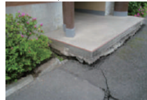
<Subsidence caused by liquefaction>
