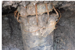
<Damaged pilings>
