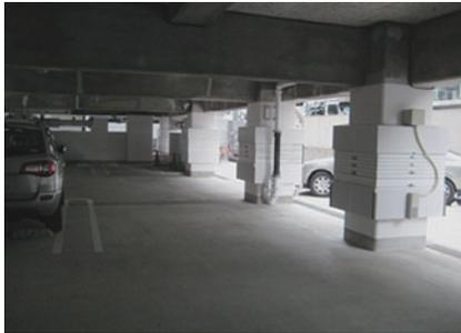
(Part of the seismic works: seismic isolation device)
